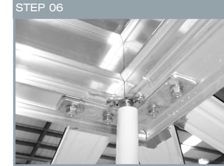
STEP 06 Assemble and fit the pre-cut tie bar assemblies. The vertical bars attach to the drop rod connecting spigot (as shown, when required).
