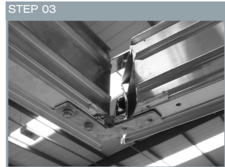
STEP 03 Also attached to each end of the eaves bottom section (when required) is a 5 way, vertical drop rod, connecting spigot.
