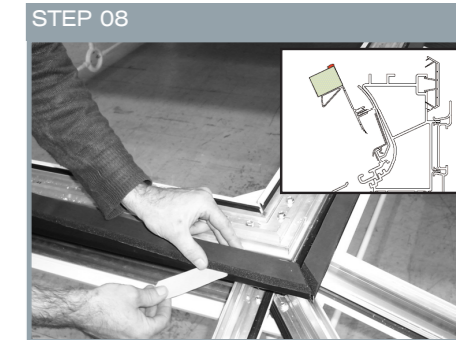
STEP 08 Apply lengths of 20mm thick close-cell-foam (supplied) to the top surface of the upper rain baffle leg, flush with rear edge (see sketch).
