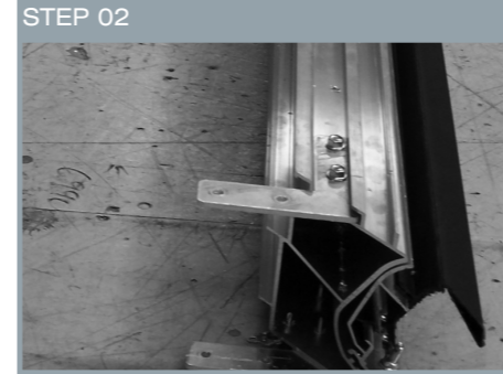
STEP 02 Each end of the lantern ringbeam (front section) will have two factory fitted 90 degree jointing cleats.
